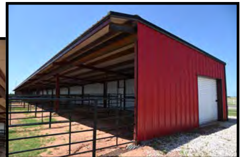
Upgrades at the Rodeo Complex
